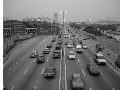
Figure 6. Freeway with a wall dividing opposite traffic lanes.
